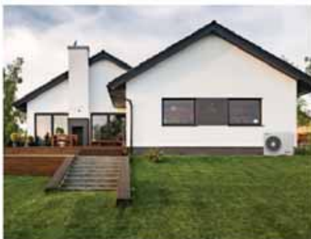
Air Source Heating
